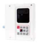
**Control of 1 cooler**, it's 230 V powered and it communicates with the board already installed in the adiabatic unit.
